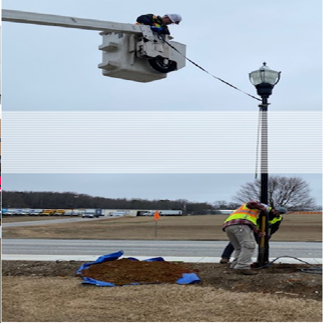
Facilities staff installing light post at Station 56.
