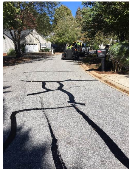
Crack Sealing in Riverside Chase
